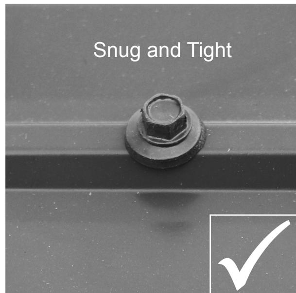
The roofing screws can easily crush the Roof Panels and Roof Edges when using a power drill. We recommend hand tightening the roofing screws so that they sit snug and tight to the roofing material.
