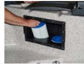
Gently unscrew and remove both filters.
